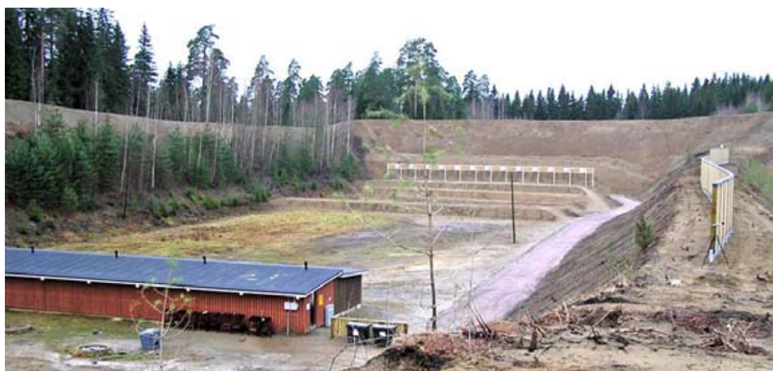
Figure 1. Parolannummi shooting range: an acoustically improved firing shed and heightened noise berms; an additional noise wall is erected on top of the dividing berm between two 150 m rifle ranges
