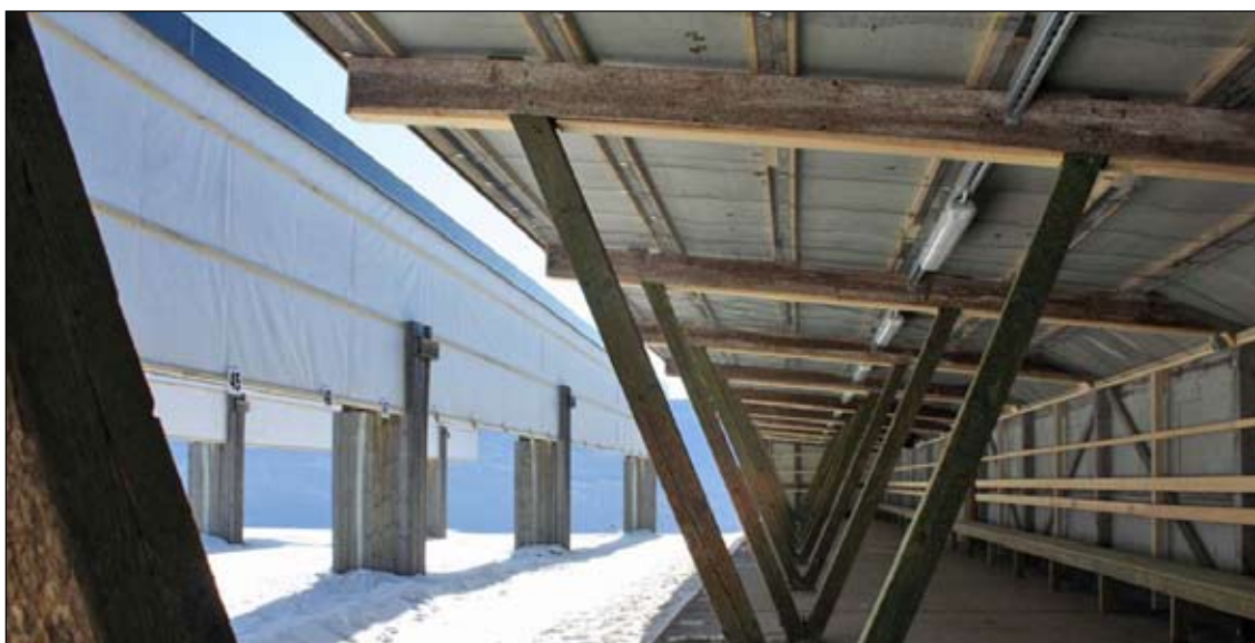
Figure 7. The original baffles at the Vekaranjärvi rifle range are lined with absorbing surface to prevent reflections backwards. Also the lower edges of some baffles will be lowered further
